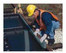
Closed-cell, polyethylene gaskets are installed to provide a seal between the Pans and rails. (Gaskets are provided.)
