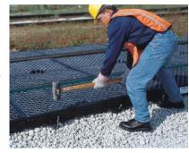
Side Pans are secured in place with 24" rebar fasteners. Typical installs require two pieces of rebar per Side Pan.
